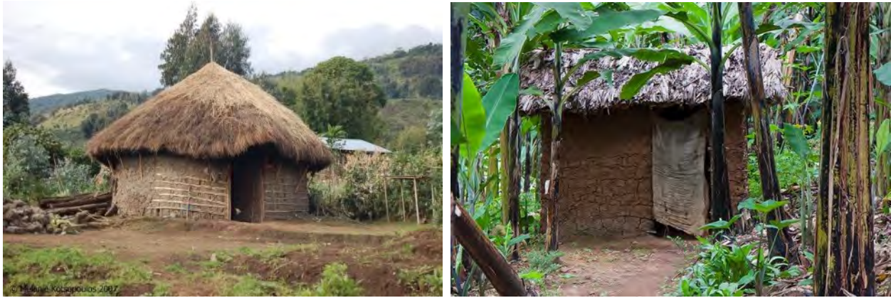
Figure 68. A house on the outskirts of Volcanoes National Park in Rwanda constructed from mud and wooden poles and thatch grass (left). A house in southwestern Uganda constructed from mud bricks and wooden poles with a corrugated iron roof (right)
